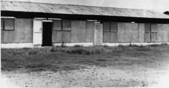
Tran Hung Dao Annex Classroom building
